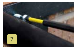
7 Align Wall Planter frame to holes and start to screw into the wall plugs. Using your screwdriver, fully tighten your screws.
