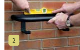
2 Using the spirit level, ensure the Wall Planter frame is level.
