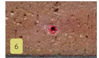
6 Place plugs into the holes.
