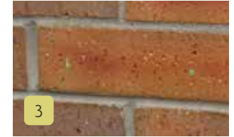
3 Mark the 4 holes in the back of the frame on the wall using your marker.
