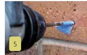
5 With your hammer drill and masonry bit, drill holes sized for your wall plugs to the depth marked on your drill bit.
