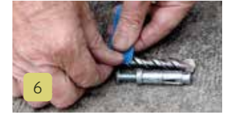
Mark your drill bit for hole depth and an allowance. Make sure that you clean the area to help ensure proper contact and make it safer to work around.
