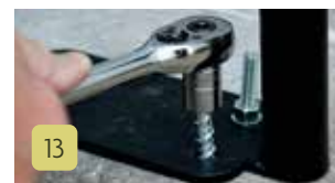
Position the base plate to allow the 'bolts' to pass through the base plate into the previously positioned inserts.
