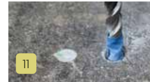
Continue to drill your holes to the depth marked on your drill bit. Clean debris away from your holes.
