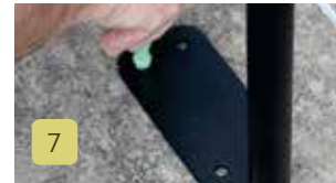
Mark holes for the base. Place the Path Light on the ground where you will install the Path Light. Mark the holes through the base with a marker.
