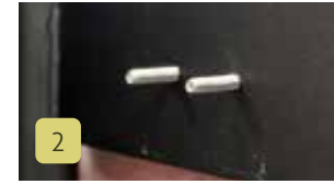
Position the 2 bolts through the fixing plate.
