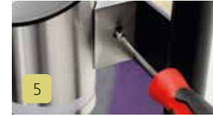
Position the solar lights over the block and using the 2 screws provided secure the light.
