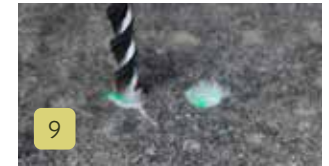
Using the appropriate drill start drilling the holes, before drilling too far check the hole alignment. Place the base plate over your hole marking and ensure your holes will align to the base plate.
