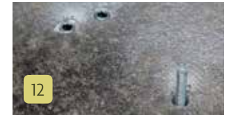
Insert into your chosen fixings (expanding bolt/resin bolt) into your four holes. If you have chosen the resin bolt fixture allow the resin to cure, with a stud in place as per manufacturers instructions.
