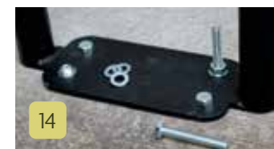
Fully tighten the 'bolts' (or nuts in case of resin bolt) using appropriate tool. If you have used a resin bolt fixture, remove the excess stud bar.
